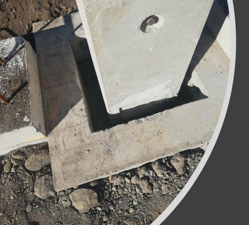
Concreting of columns to footings
