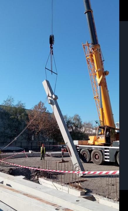
Positioning the pillars vertically by a crane
